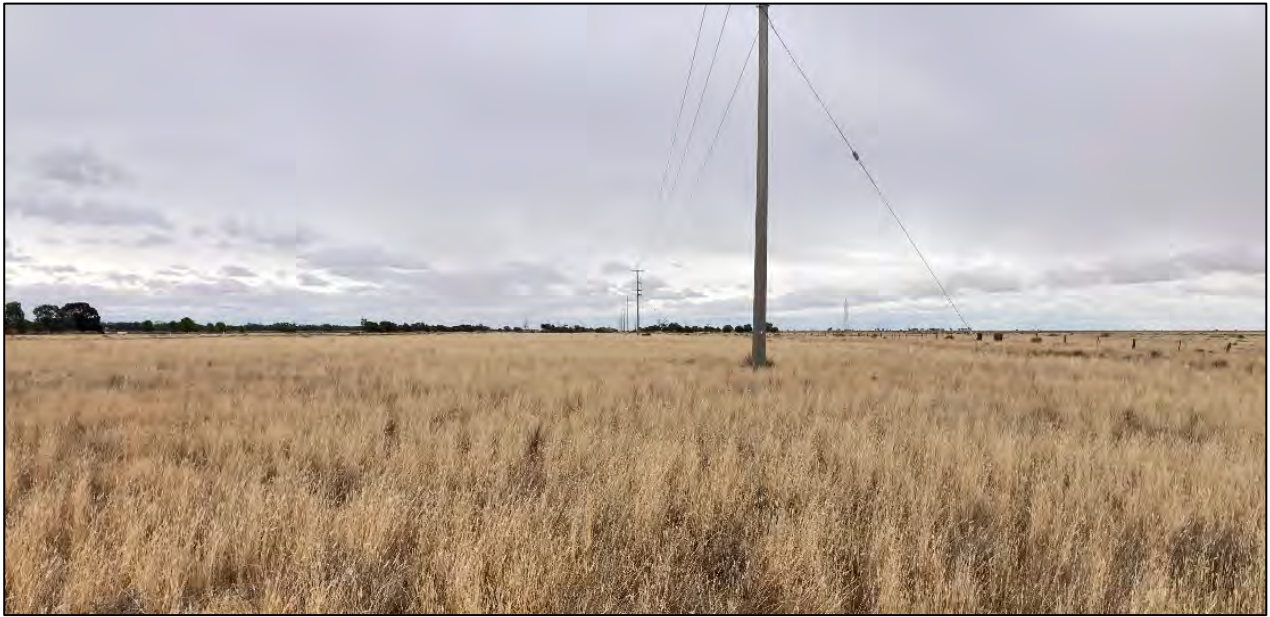
Photo 4: Existing power line infrastructure within the study area and immediate surrounds. Photo: D. Wall, 2024.
